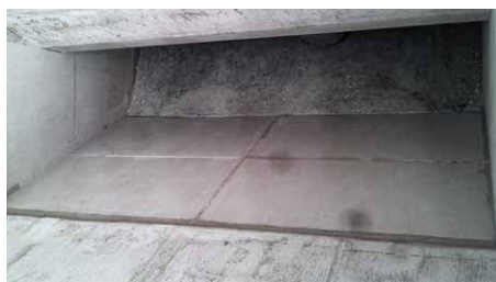
\ Ramp and nose beam – precast piece Rampa y nariz torre fusora
